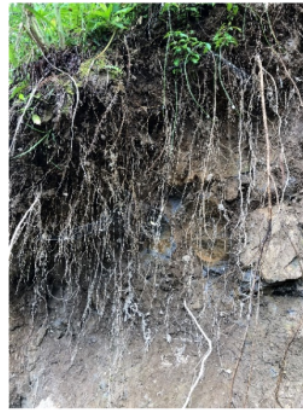
Figure 6. Plant Roots in Landslide Field (T2)
